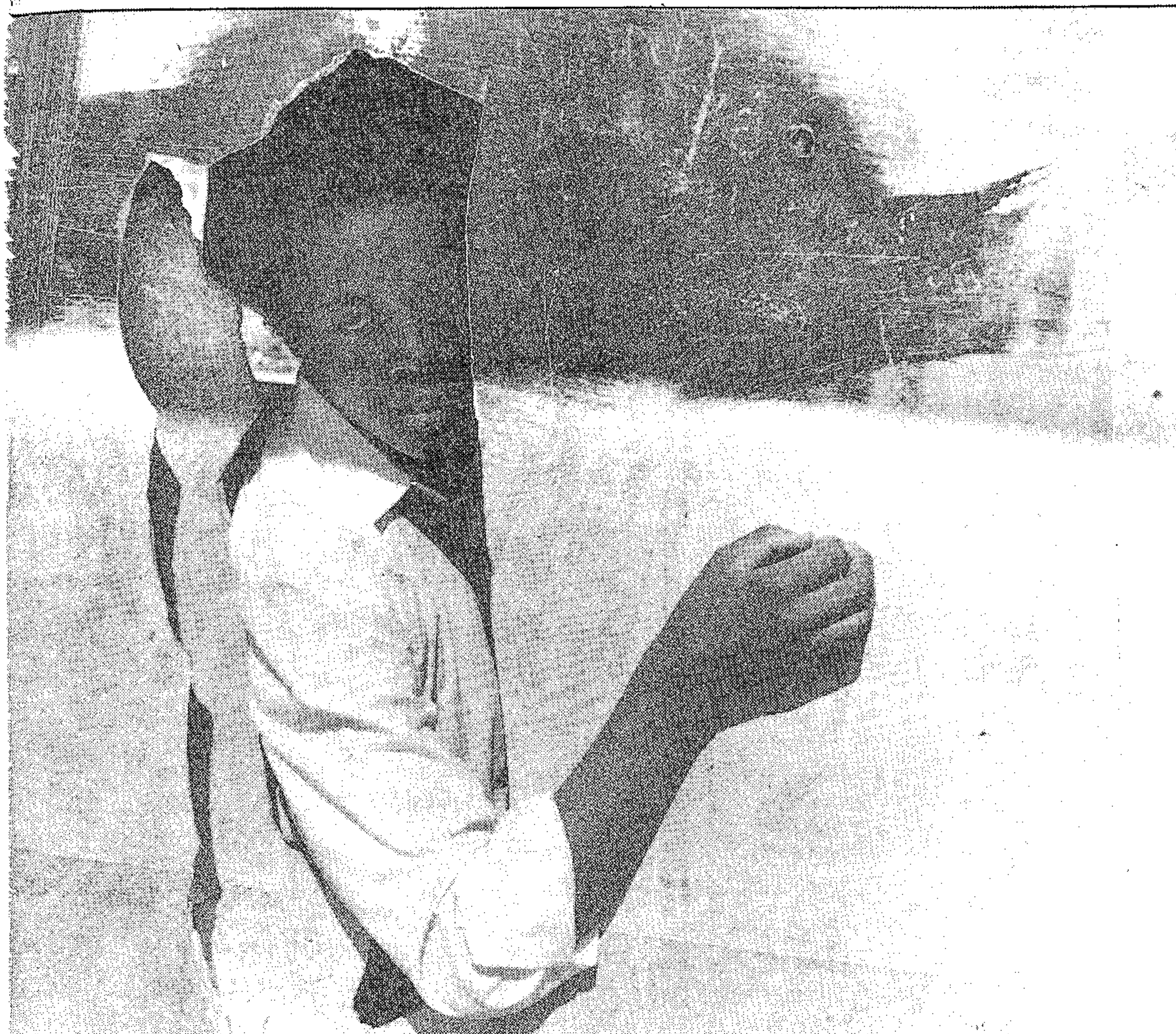
Showing the scars . . . Hlengiwe Secondary School pupil Constance Tsekedi (above) peers through a gaping hole in a classroom wall. Wellington Mokone (left) points to gaps in a roof damaged during unrest. Pictures: George Mashinini
