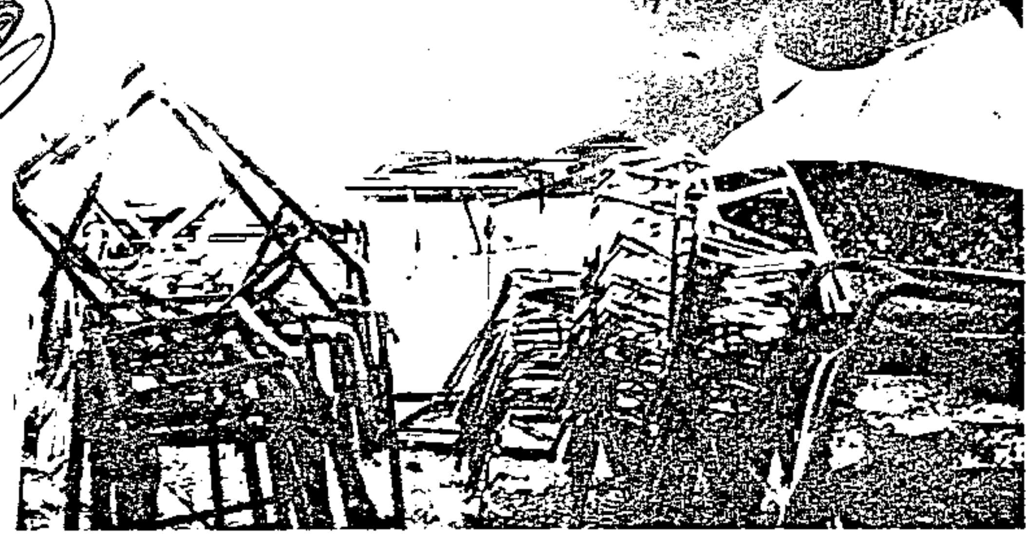
A pile of burnt desks in a damaged classroom at Fezeka
