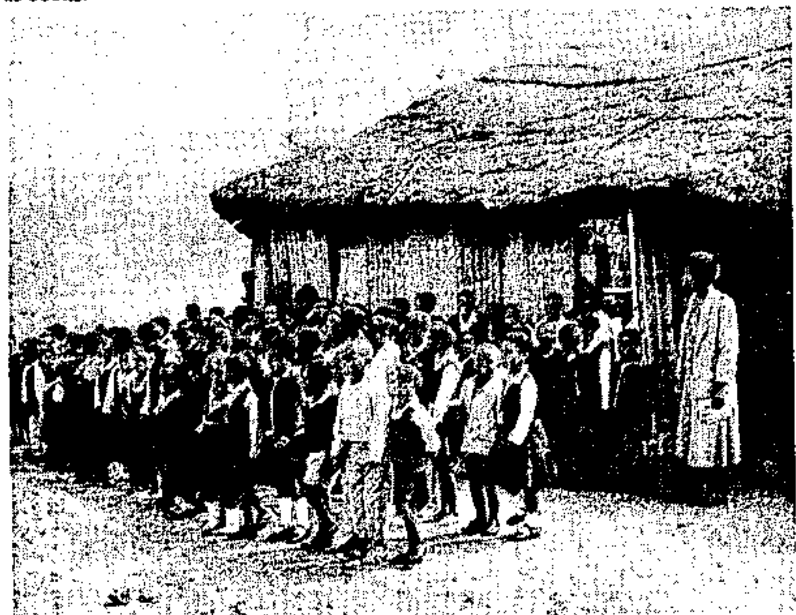
The exterior of the Sweetwaters squatter camp school. It is poorly constructed and the children will suffer badly during the coming cold winter months.
