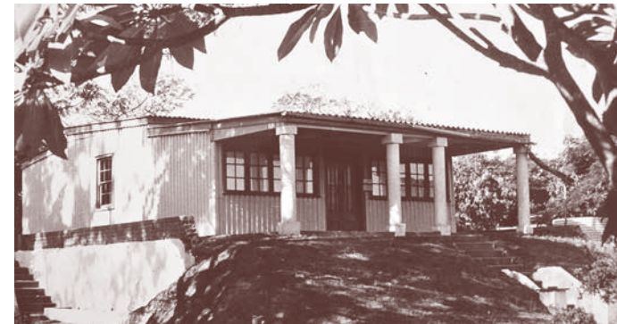
Sarvodaya in the 1930s. The corrugated iron sheets were later replaced by asbestos sheeting
