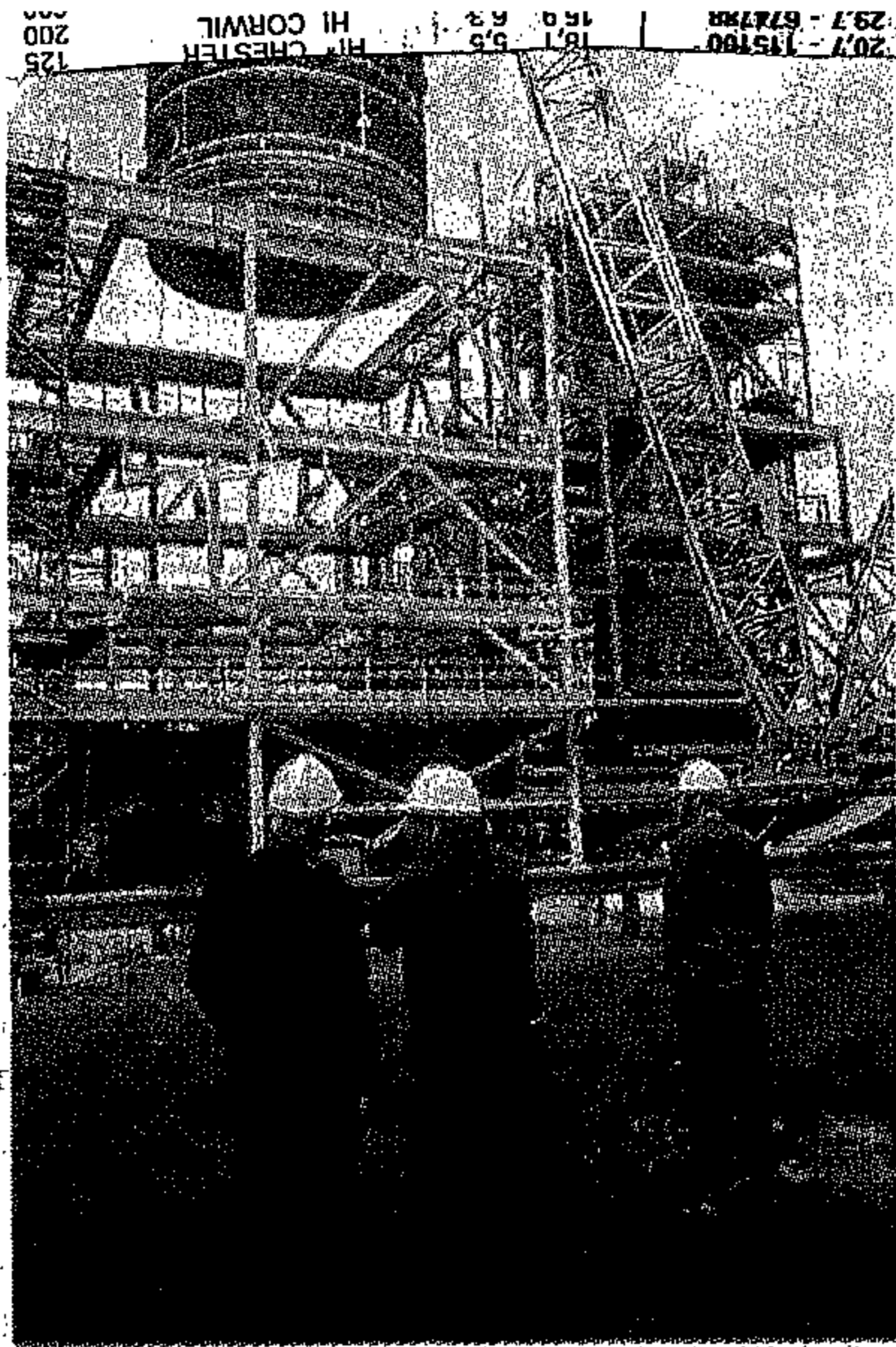
GETTING A LIFT ... the new-generation Sasol advanced synthol reactor vessel being hoisted into position at the Secunda site of Sasol Synthetic Fuels.
