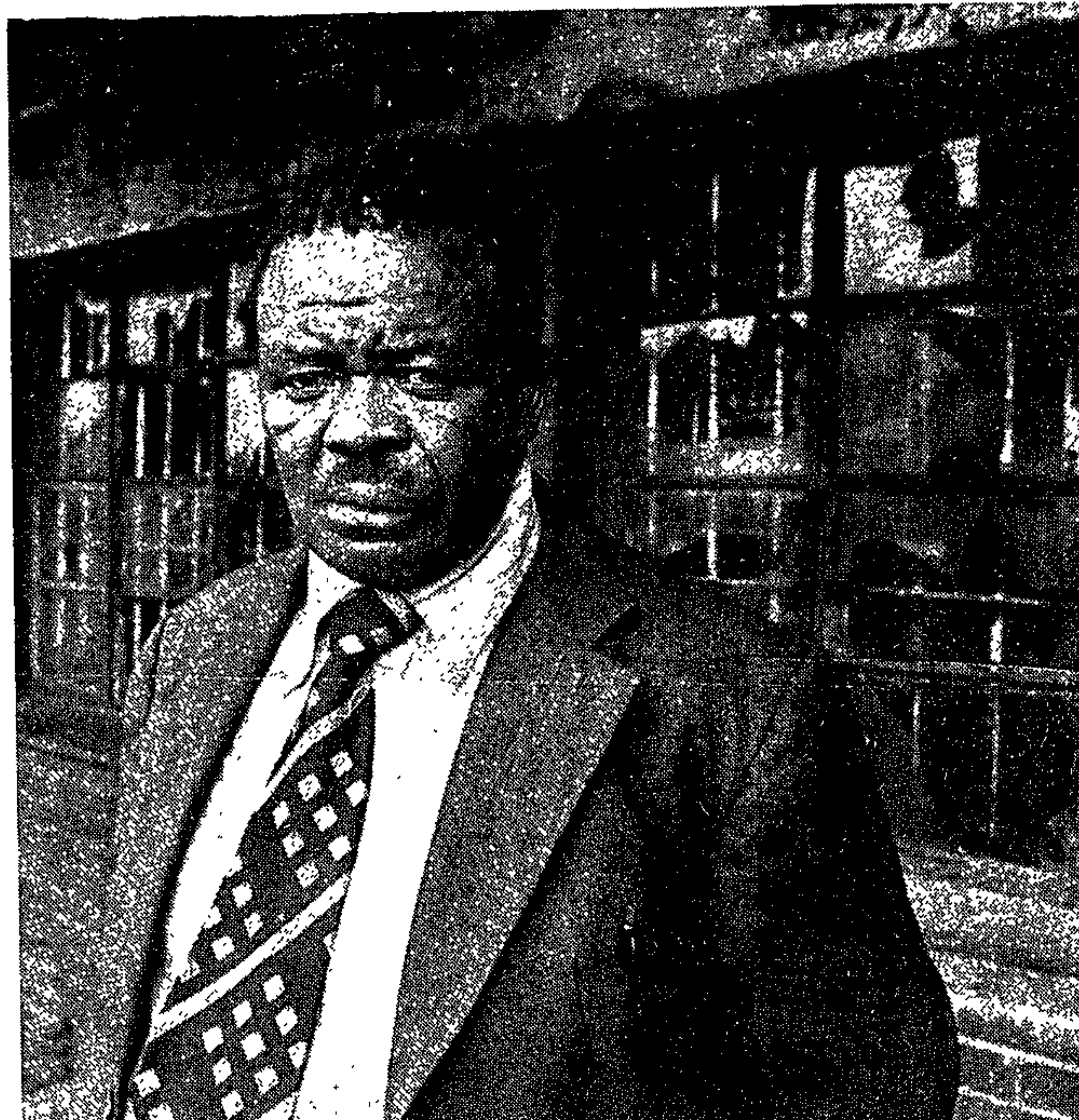
Mr Shadrack Mtetwa in front of his demolished shop.
