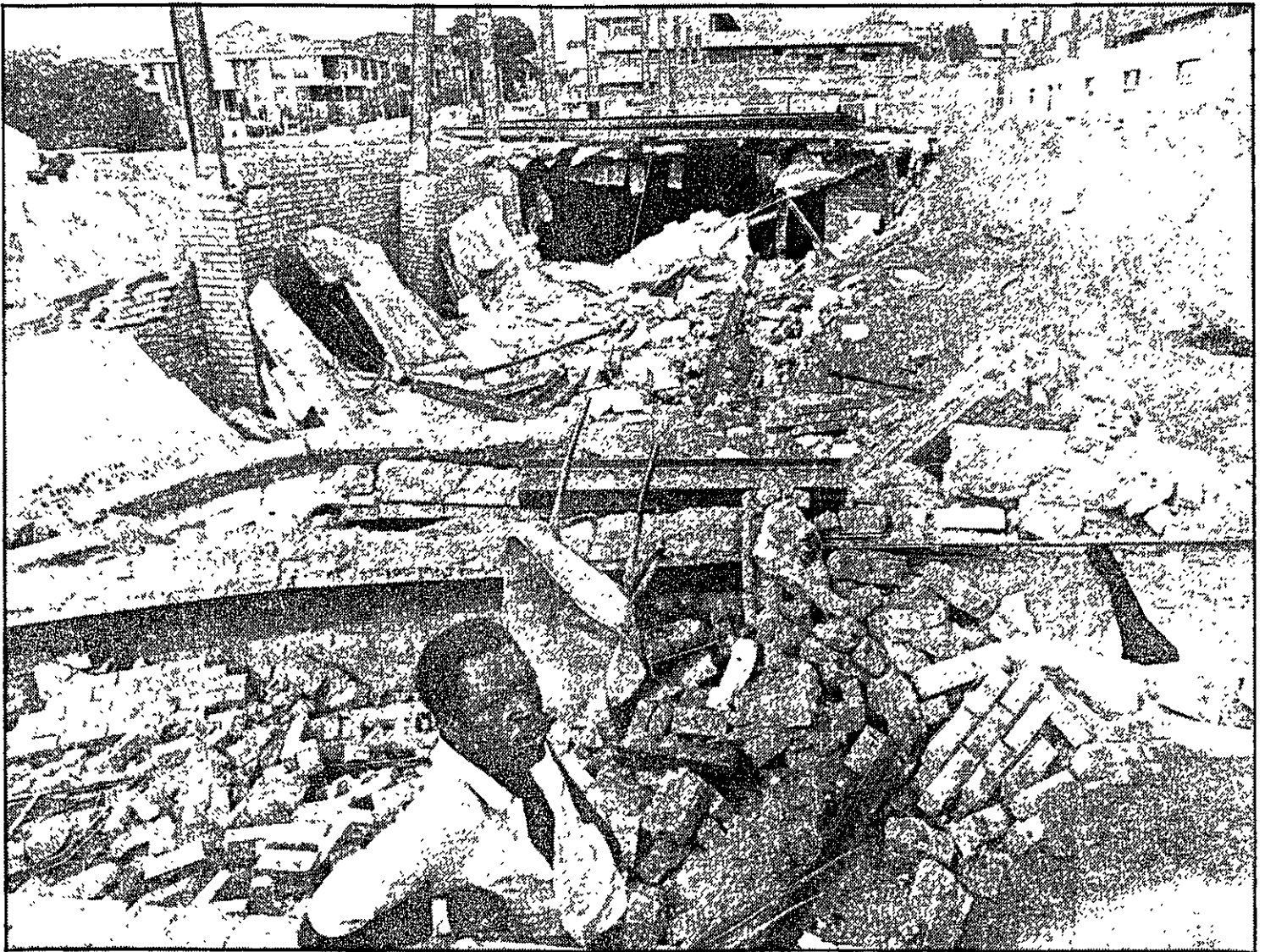
Building site tragedy . . . a worker stands in the underground parking area of the Ferndale office complex shortly after a 100 sq m section of roofing collapsed, killing a man and injuring four. Picture: Jacob Rykliff
