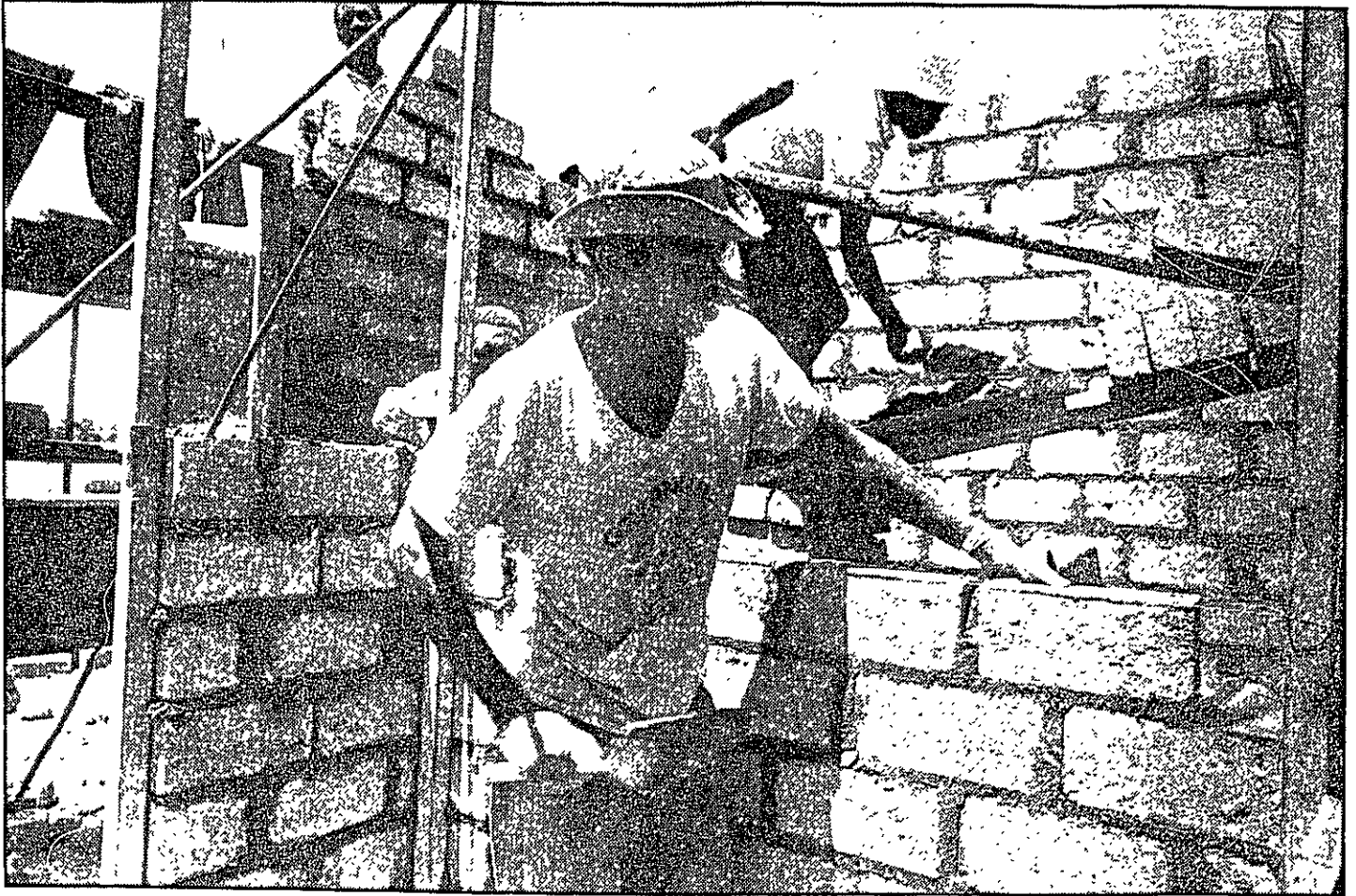
Rush job . . . bricklayers Rufus Malaje and his teammates rush to complete the building of a house at a site in Lenasia so that they can collect their meagre wages. Picture: Ken Oosterbroek
