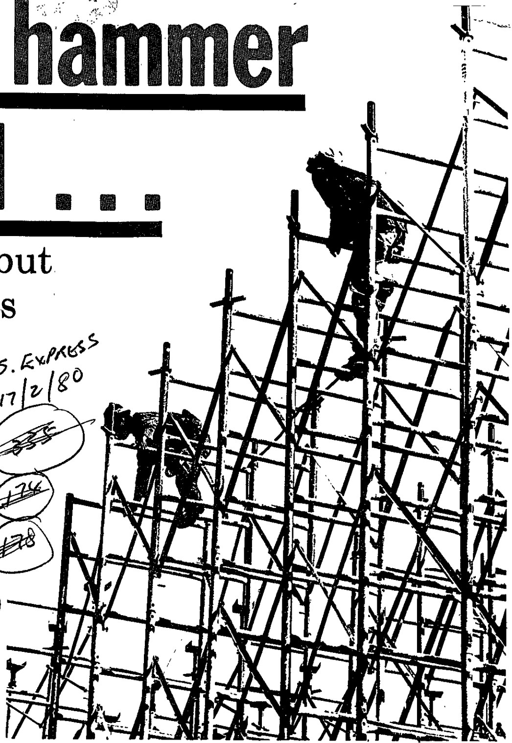
● Workers atop the scaffolding . . . a head for heights is an advantage.
