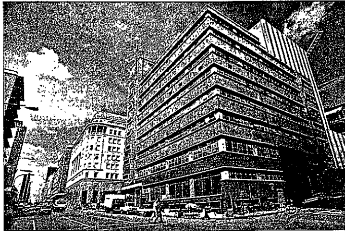
Auto House ... out of implosion, bricks and work
