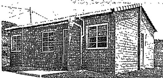
BRICK HOUSE: A three-bedroom showhouse built with single-skin walls in a township near Tongaat in Natal.
