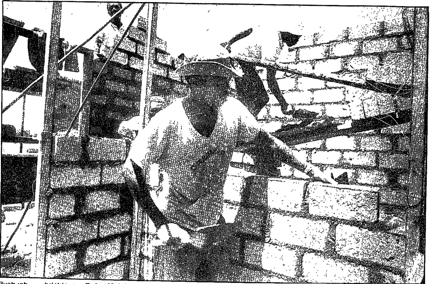
Rush job . . . bricklayers Rufus Malaje and his teammates rush to complete the building of a house at a site in Lenasia so that they can collect their meagre wages. . . Picture: Ken Oosterbroek
