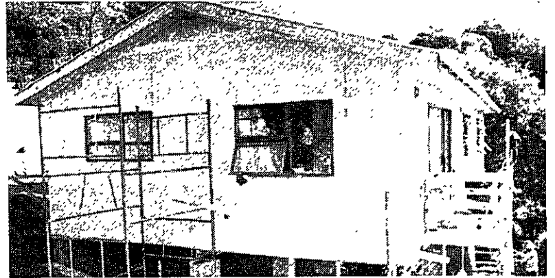
□ A timber-frame house under construction
