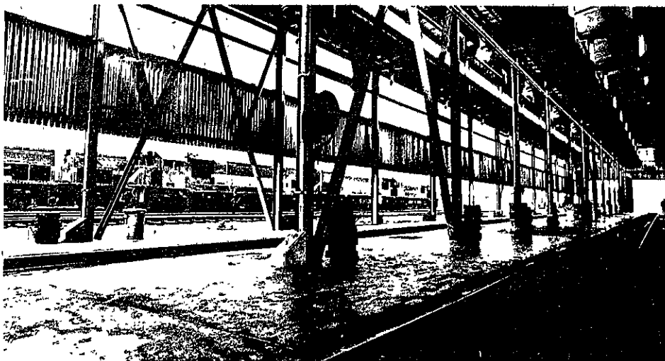
The diesel locomotive maintenance depot at Richards Bay . . . built by Roberts
