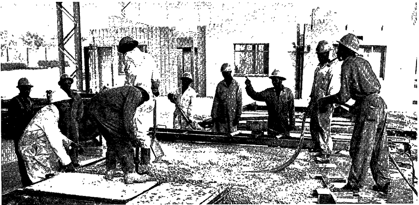
Casting concrete components at M&S's Philippi factory
