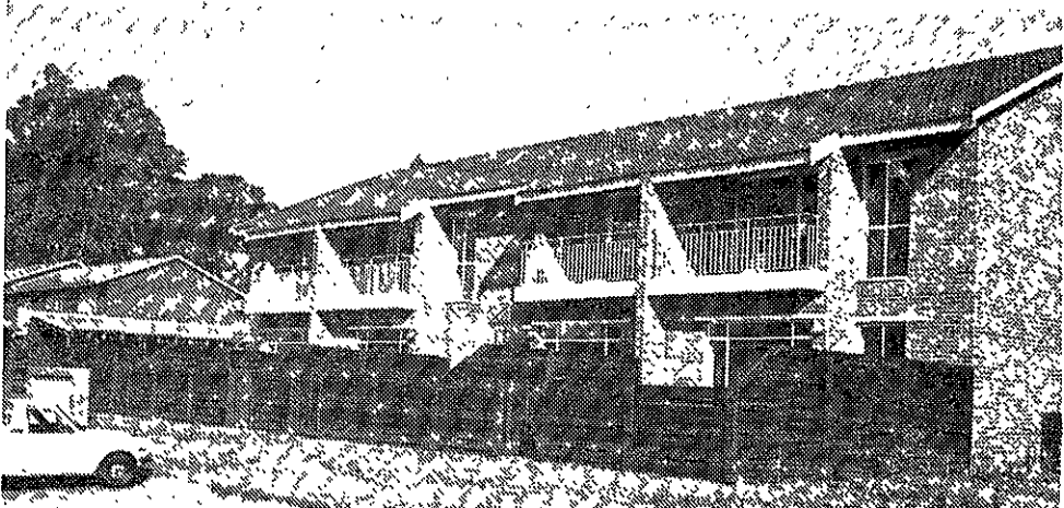
ROBERTS Construction Property Developments have completed and handed over their latest 15 town-houses. The project, known as "The Firs" (above), is in Bedfordview and consists of 15 duplex town-houses. All were handed over on due date. The development was fully let three months prior to the completion.
