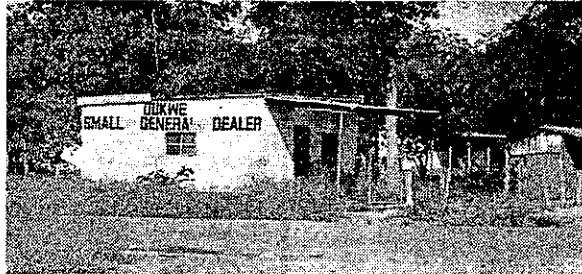
DILAPIDATED ... this small grocery store is a symbol of the decay at Dukwe. Picture: JOE SEFALE
