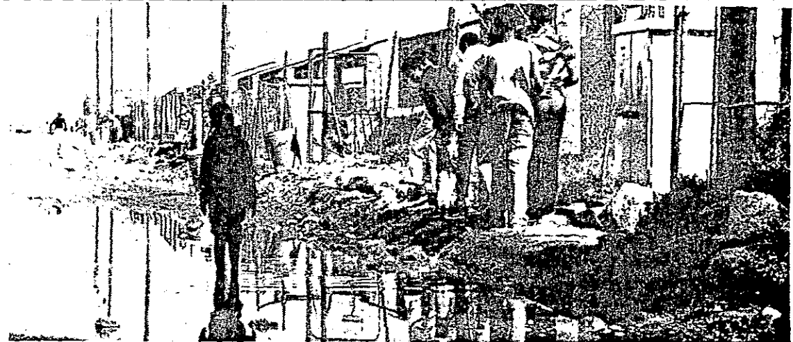
SEWERAGE PROBLEMS: The pool outside house number 1432 Mofolo North.
