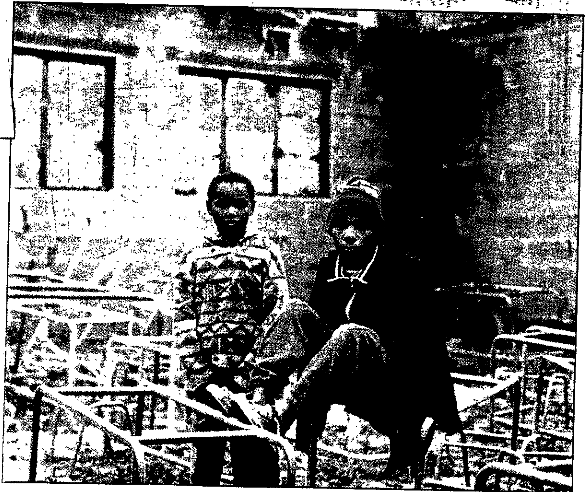
Brothers Monk (standing) and Awu Motaung, pupils at Caledonia Primary School near Ficksburg, stand inside the charred remains of what used to be their school. Yesterday they were sent home because the cold weather made it difficult to study outside.
