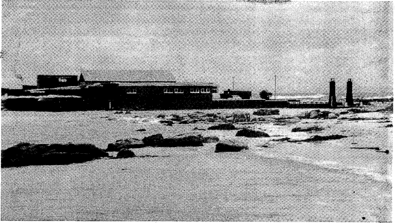
INSTANT ISLAND — JUST ADD WATER: The narrow channel on the right of the picture was enough to make the Soetwater site an island — and legalise the fish factory
