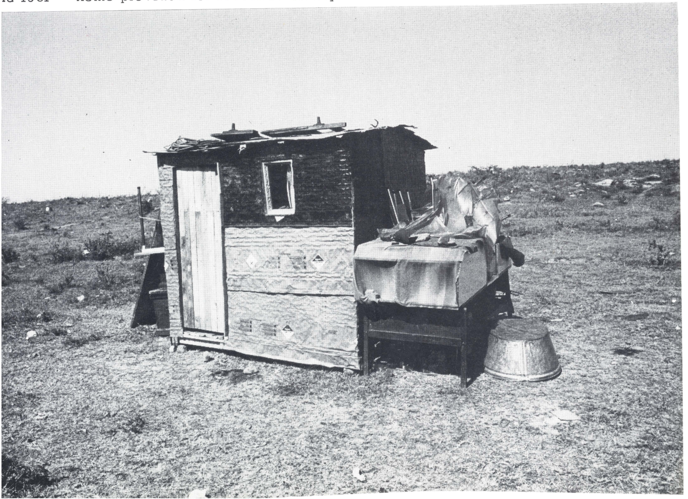
na 1981 - home provided for resettled family
