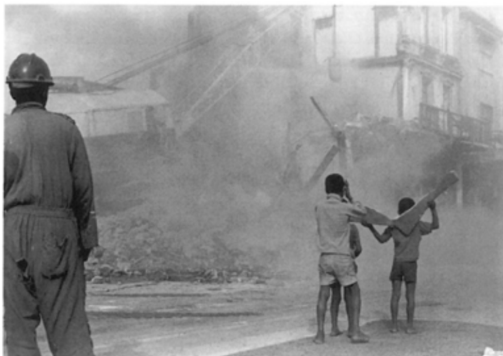
Demolition, District Six Paul Alberts
