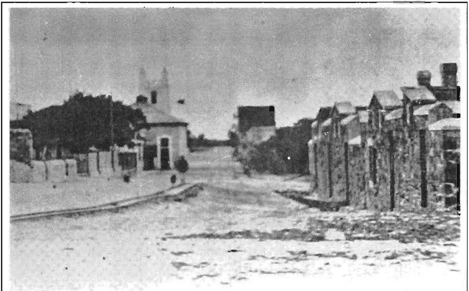
The main street on Robben Island. Anglican Church, water tank. Two mules walked in a circle all day to pump water up.
