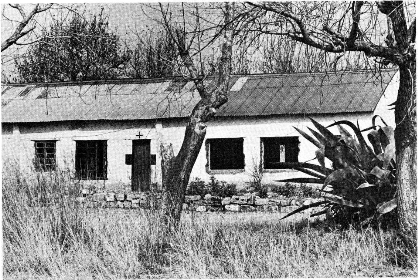
Bultfontein school now derelict three years after it was closed.
