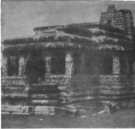
Aihole, in the Bijapur District of Karnataka, cradled the Chalukyan style as Mahabalipuram did the Dravidian. The Temple of Durga is interesting as a Brahmanical adaptation of the architecture of a Buddhist Chaitya with an apsidal end.
