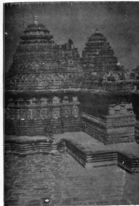
The Kesava Temple at Somnathpur (13th century) is a typical example of the fully evolved Hoysala style. It is a three-celled structure with a tower on each sanctum.
