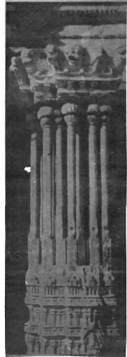
Among the more interesting parts is this monolithic "musical pillar". Each of the shafts in this composite pillar when struck with a rod yields a distinct musical note.
