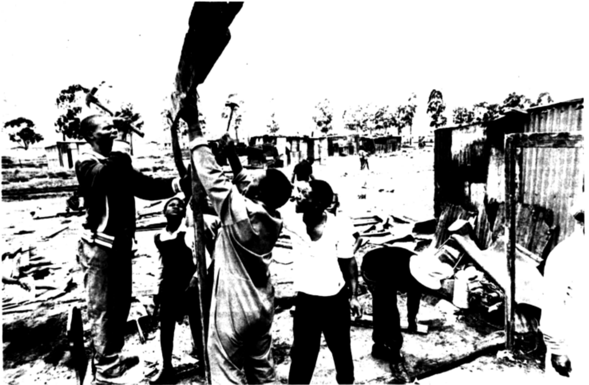
Residents in Silverton, Tsakane rebuild shacks which had been pulled down by the East Rand Board
