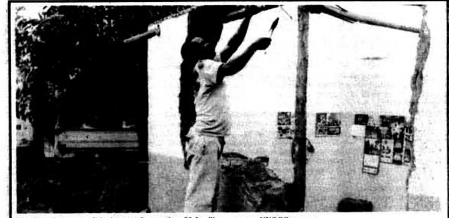
Breaking down one of the houses of more than 80 families forcibly removed from Uitvlugh village. Moutse, to Immerpan. The Uitvlugh youth congress (UYOCO) condemned the removals saying villagers had lived there for more than 20 years and are resisting the move. They said government officials paid some individuals to recruit more people to move to Immerpan and were trying to
