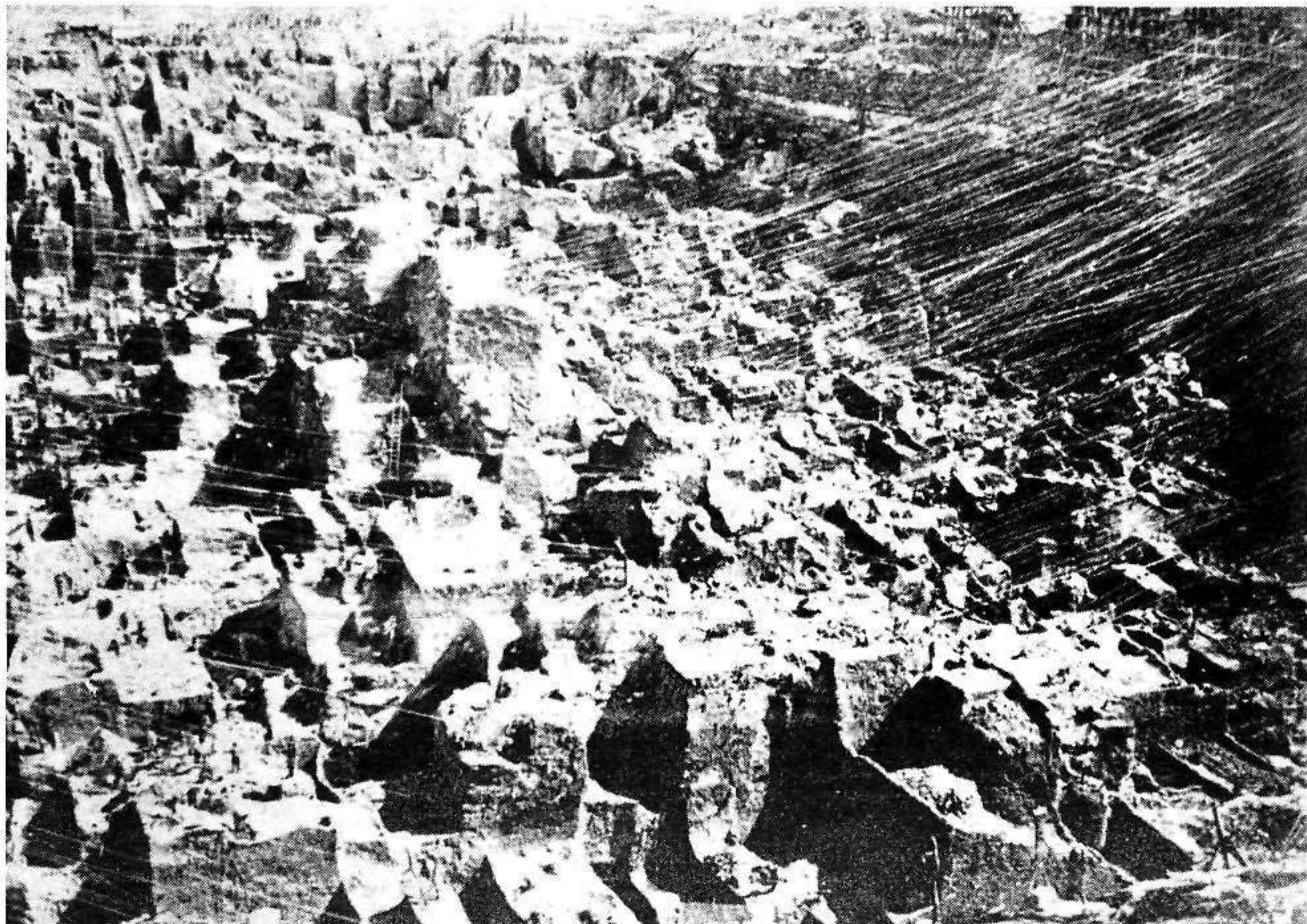
The Kimberly diamond mine. Each prospector owned a small plot which he dug with the help of African labour. The plots were linked to the surface by a line which was used to haul the dug rock to the top where it was then sifted for diamonds.
