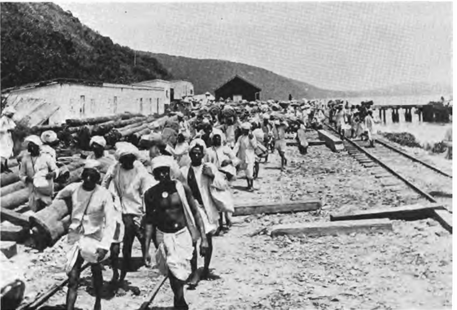
10. Crossing the railway line on the way to the Bluff.
