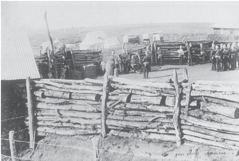
Fort Curtis constructed in October 1883 by the men of the Eshowe Column. The timber stockade, which was commanded by an earthwork lunette, is shown in the photograph with men of the garrison and a 7-pounder gun. Photo INIL 7583 courtesy of the National Library of South Africa (Cape Town campus).
