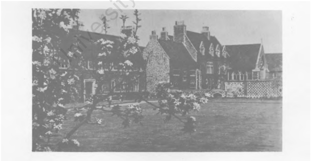
18. St. Augustine's College, Canterbury - the Native Building is in the centre.
