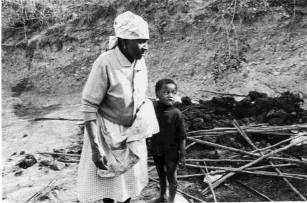
Mrs Ngubane outside her home, which was demolished by state officials.
