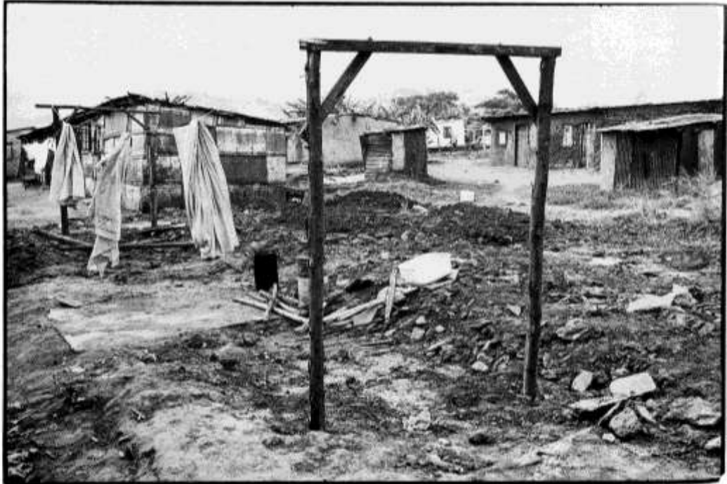
Recently demolished houses, Amouti.
